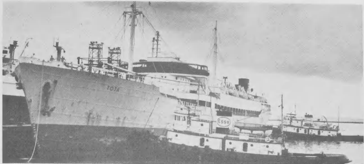
THE TOTA is a transport ship that serves the whalers in their Antarctic hunting grounds. It is a tanker with accommodations constructed above deck. It carries fuel oil south and whale oil north.
